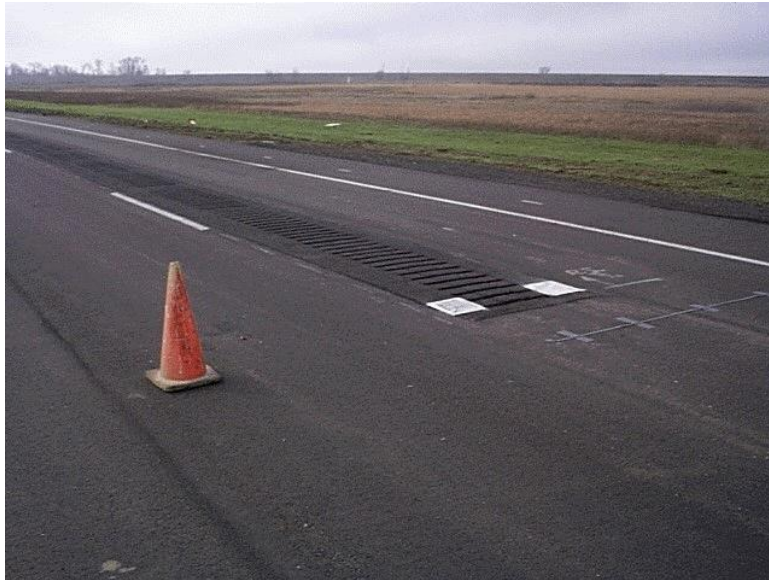
Gambar 9. Rolled Rumble Strips
