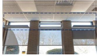
Gambar 2.21 Reflector light shelf Sumber : https://www.dattner.com/projects/view/bronx-library-center/
